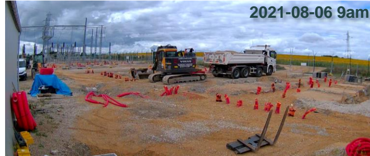
TONNERRE PROJECT, FRANCE
