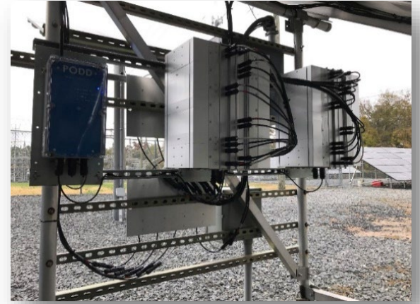
Alencon SPOT DC/DC String Optimizer (image courtesy of Alencon)
